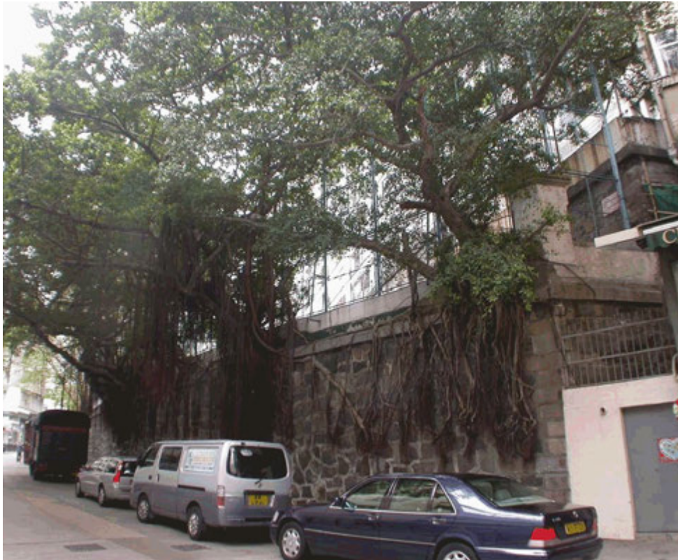
Photo 2: Retaining Walls & Trees along Hollywood Road
